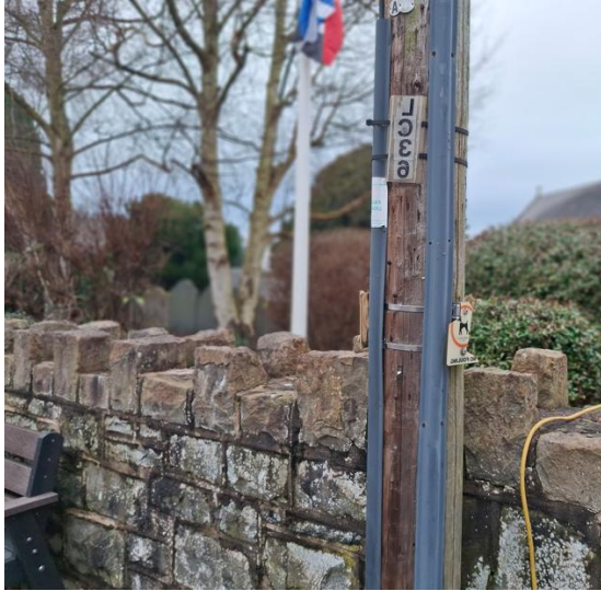
Wall at telephone box end
